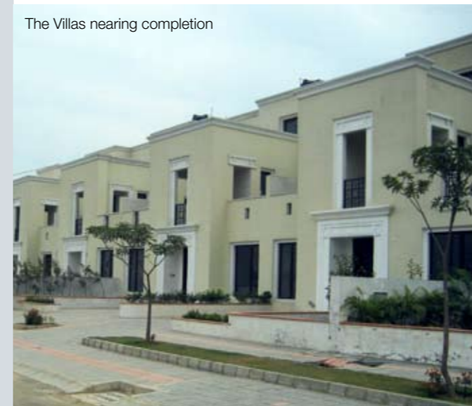
Infrastructure and Parks under development
