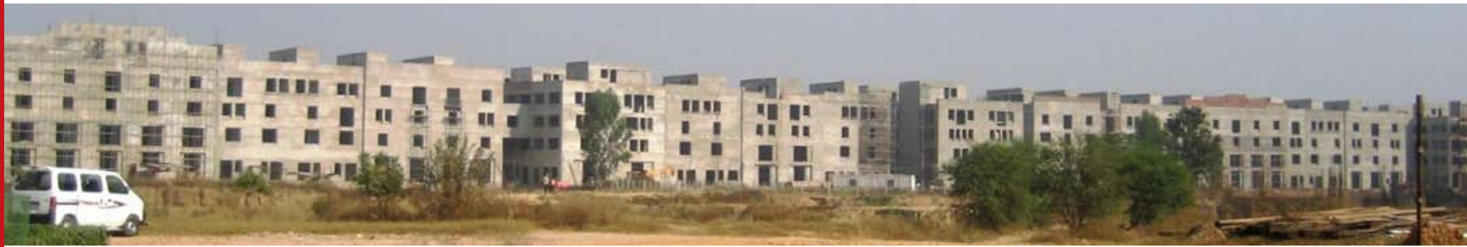
Actual shots of construction at site
